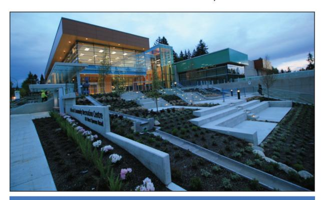
The new Delbrook's design is inspired by light and our natural environment with lots of glass and wood. The building is uniquely situated on a slope that goes from the northeast corner down 10 metres to the southwest corner. Interior spaces have been configured to maximize light and views out to the park land south of the building. An alternative solution was developed which permitted extensive use of glue laminated timbers in a main public area.
