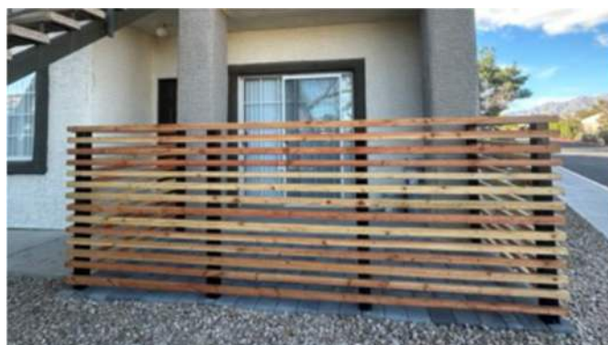
PATIO EXTENSIONS UNDERWAY, ~30% RETURN ON INVESTMENT
