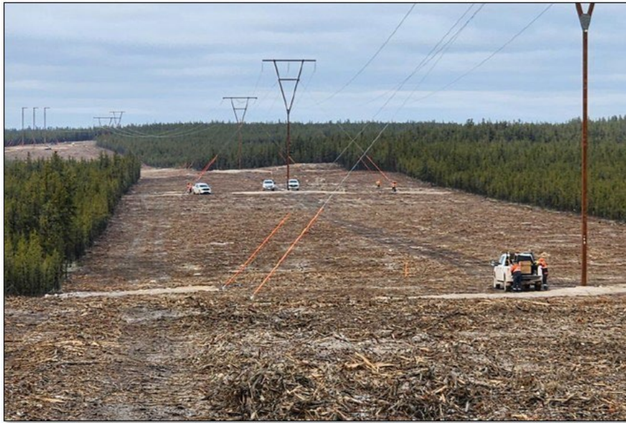
Figure 1: New SaskPower 138kV Transmission Line to the Site of the Future Phoenix Uranium Mine
