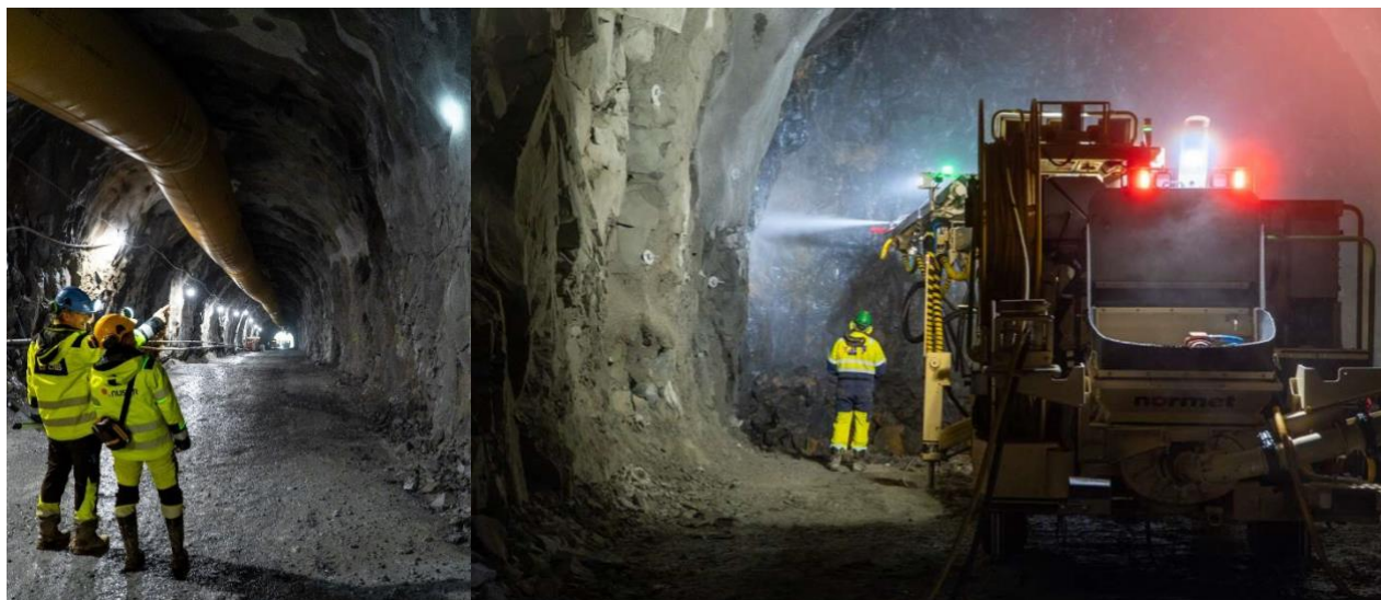
Figures 1 & 2: LNS and Blue Moon advancing underground development at Nussir (inspecting tunnel wall left and ground support activities at the face right )
