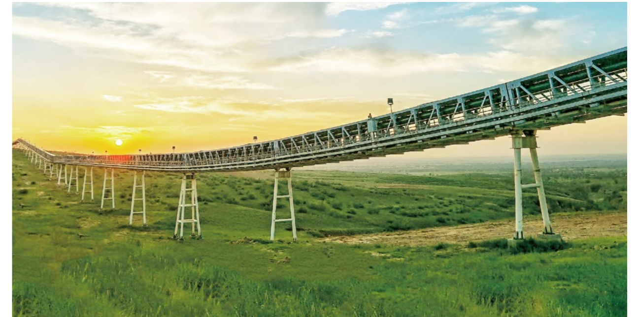
During the implementation of the small watershed comprehensive governance project for the Kūlietu Stream, Inner Mongolia Tuoketuo Power Generation Company has utilized pipeline transporters to securely transport coal ash produced by the power plant to the Kūlietu Stream watershed for storage and ecological treatment. This initiative has established a precedent in China for the comprehensive governance of small watersheds using coal ash.
