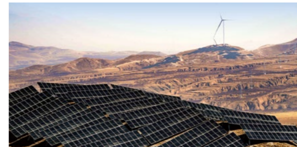
The 1GW large-scale wind and photovoltaic power project situated in Yuxian County, Hebei Province
