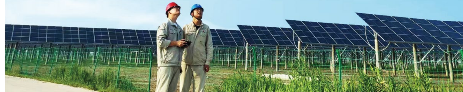
Hebei Chengde New Energy Business Unit uses drones for smart inspection
