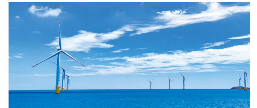
The 15 wind turbines in the Changjiang'ao wind farm have successfully completed the 240-hour trial operation, meeting all assessment criteria.
