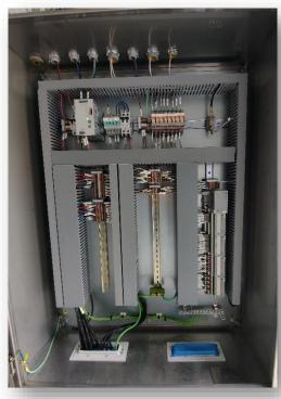
TTS integrated the new system into the customer's Allen Bradley control system. The system utilized TTS standard logic blocks for water injection that were modified for this purpose. The control's I/O was expanded using fiber optics to the new junction box and integrated into the existing ControlNet bus. TTS provided a new HMI interface screen that displays critical operating parameters. This screen was integrated into the original Wonderware HMI.
