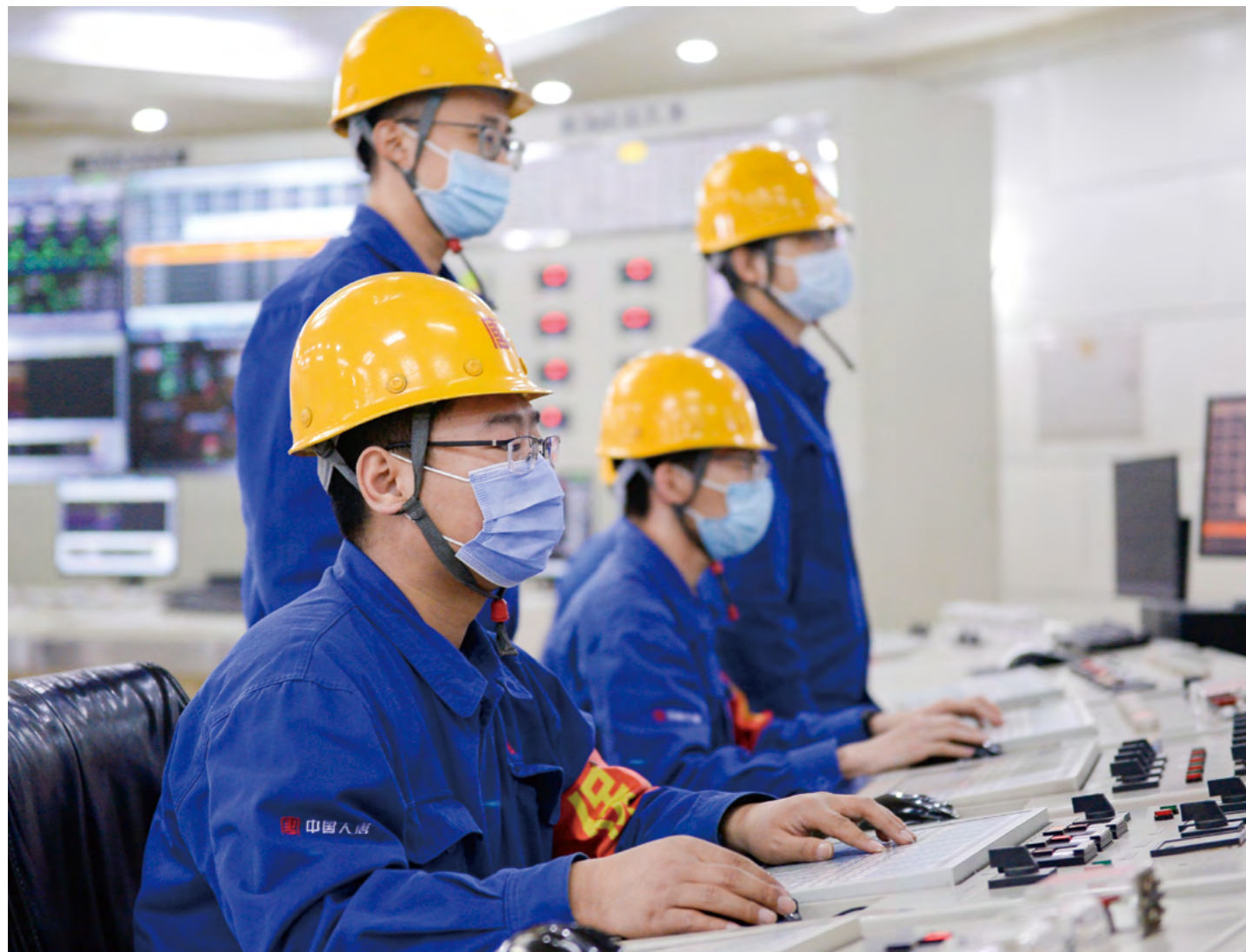
Douhe Power Plant has created a new record of safe and stable operation lasting 6,836 consecutive days.
