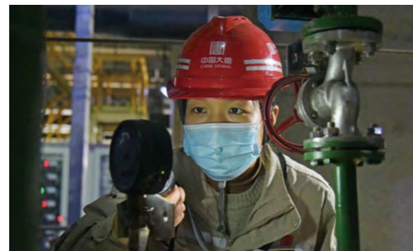
Hebei Matou Power Plant improves the maintenance of environmental facilities to ensure that their environmental parameters meet the standards.
