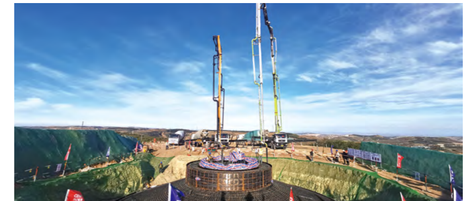
The construction site of Qingshuihe New Energy Project
