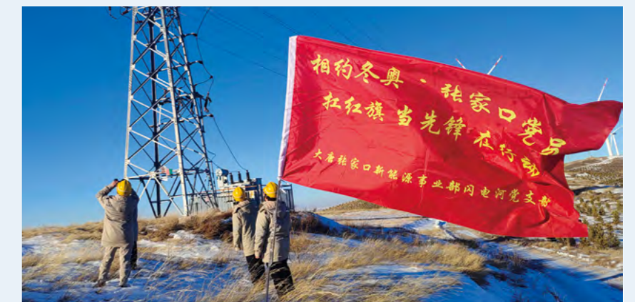
The inspection team consisted of Party members from the Hebei Zhangjiakou New Energy Business Unit inspect wind turbines.
