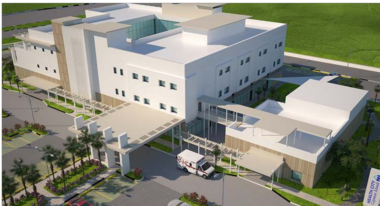
Health City Cayman Islands began construction on a new hospital facility south of Camana Bay off the Esterley Tibbetts Highway. The 70,000 square-foot US$100 million project will provide several medical specialties not yet available in the Cayman Islands including neonatal intensive care and robotic surgery (Image courtesy of Health City Cayman Islands).
