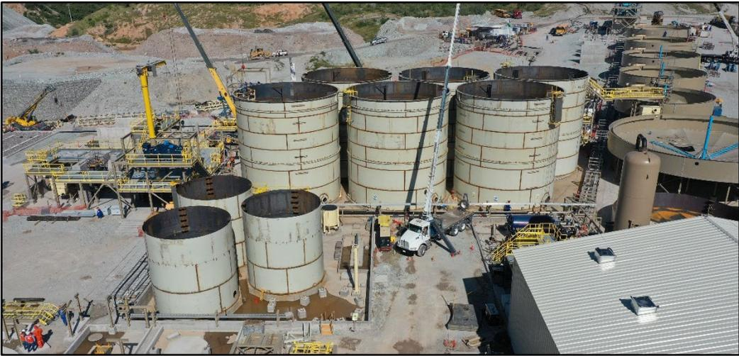
**Figure 4: Leach Tank Construction**
